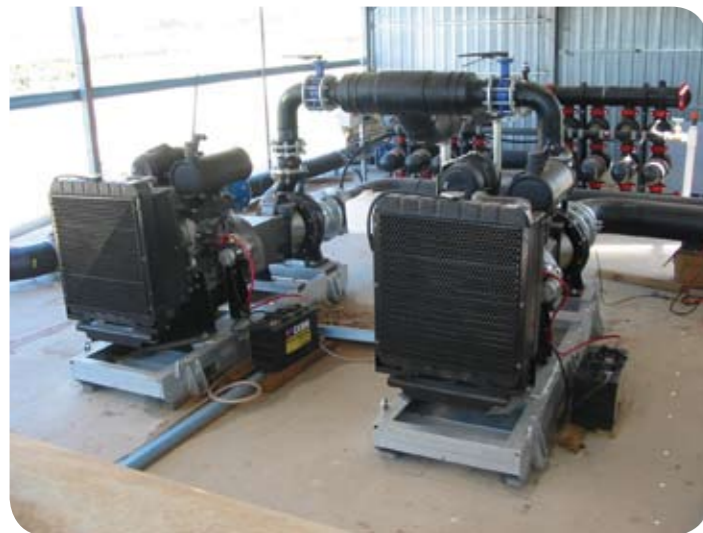
The twin Yanmar's are rigged to drive Davey ISO pumps to help protect the Tilbrook family vines
