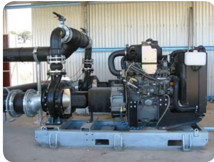
Each Yanmar 4TNE delivers a max output of 68hp from a direct injected, 3.3 litre 4 cylinder
